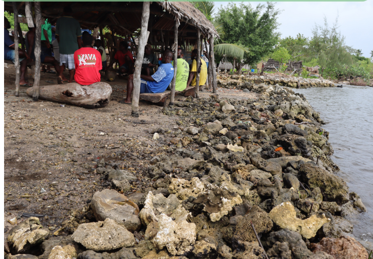
A stone wall on Maskelyne Island to prevent the sea from reaching this meeting house.
